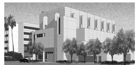
Updated concept for energy plant showing the latest noise mitigation design features (facing north from Waldemere Street). The cooling towers, which contain oversized, variable-speed chiller fan blades, will be enclosed on four sides at the top of the 90-foot-tall structure. The size of the fans and the enclosure adds height but reduces sound.
